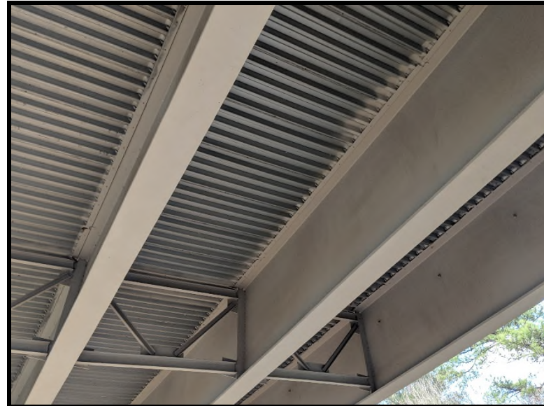
2 View of the metal deck and metal support beams.
