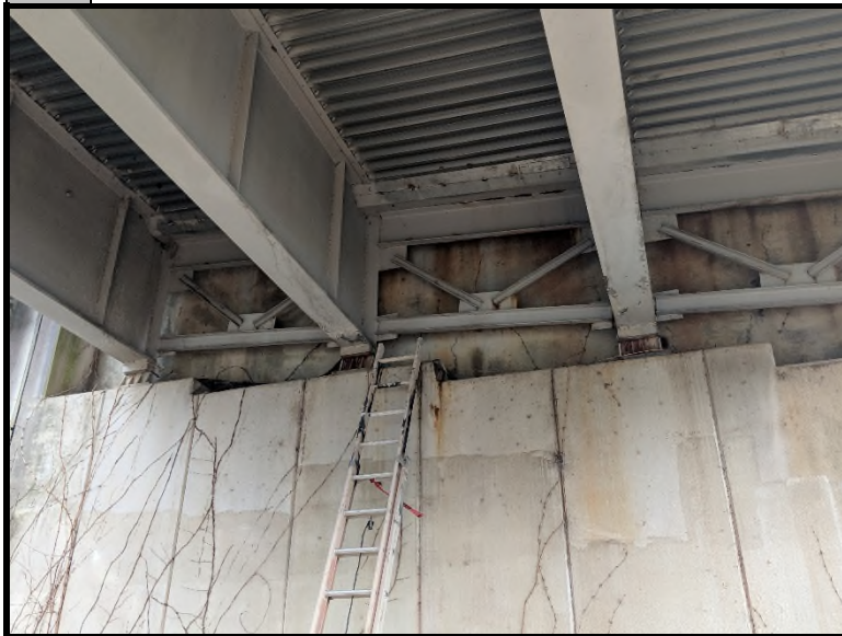
3 View of the underneath of the foot of the bridge.
