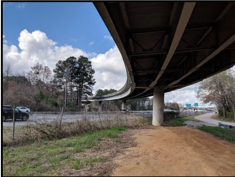
1 View of the I-126 Westbound bridge to I-26 Eastbound.
